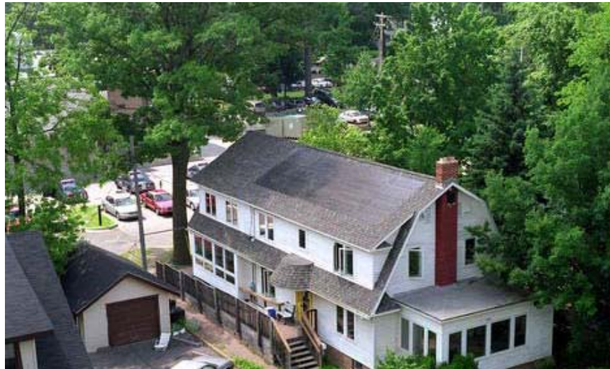
Figure 5. A SOLAR PV ARRAY SURROUNDED BY MANY TALL TREES THAT CREATE SHADE ON THE ARRAY DURING THE DAY.
