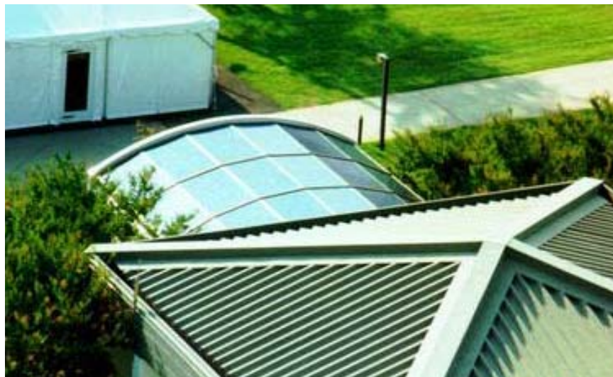
Figure 4. A SOLAR PV ARRAY CONSTRUCTED AS A BUILDING ENTRY, GIVING AN EFFECT SIMILAR TO THAT OF DIFFUSE SHADING.
